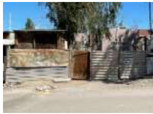
Image 3: Fences made from recycled zinc galvanized roofing.
