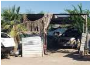
Image 4: Doorways made from recycled zinc galvanized roofing.
