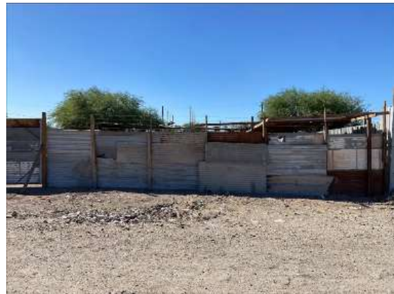
Image 2: Recycled steel roofing sheets.
