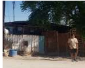
Image 4: Doorways made from recycled zinc galvanized roofing.
