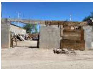
Image 5: Entryways made from recycled wood and homemade stucco.
